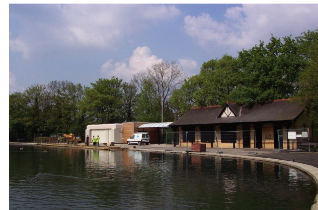
Refurbishment of Boathouse and Lakeside Cafe in 2006
