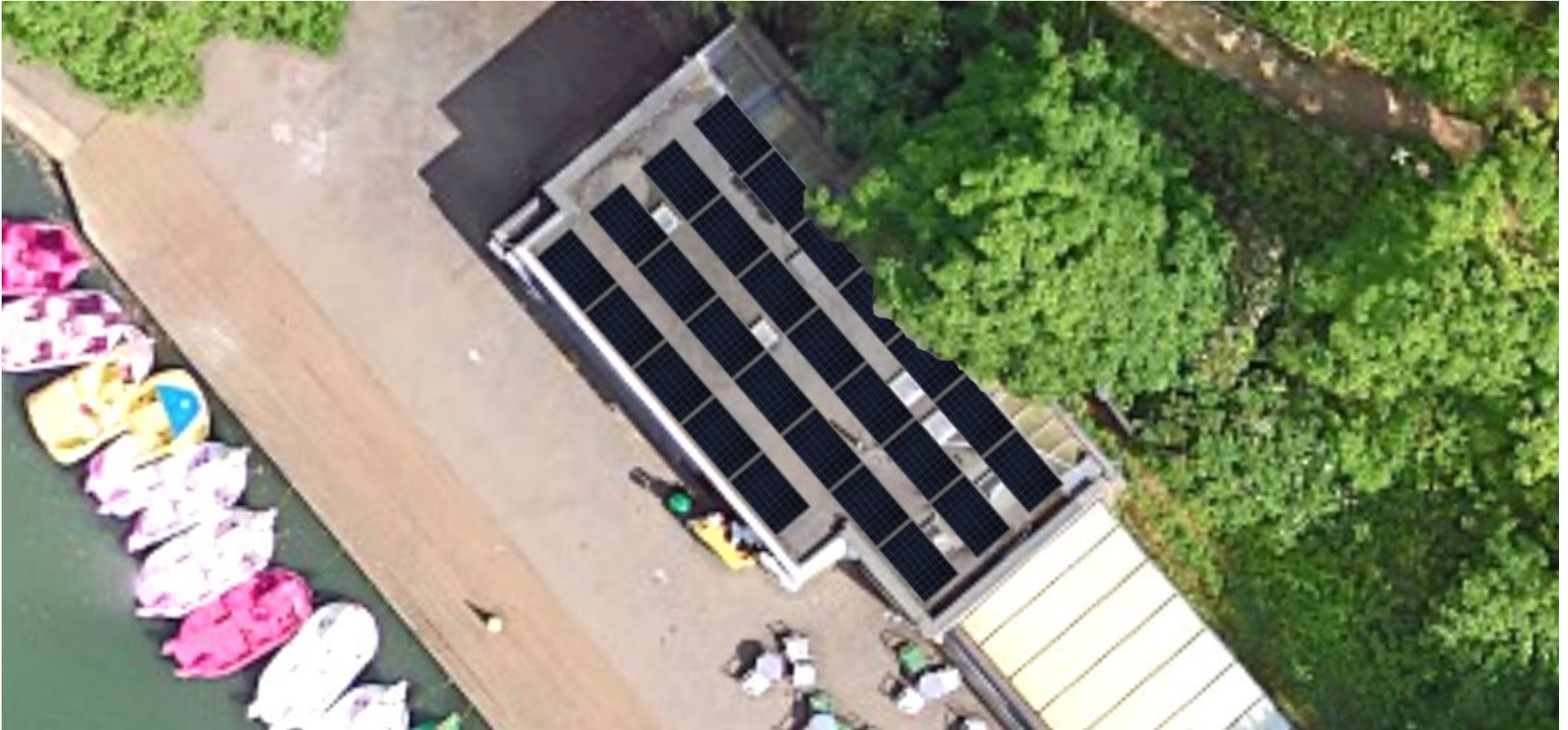
Solar Panel layout on boathouse roof.
