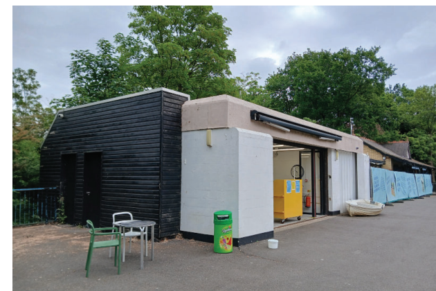
Boathouse southwest facing frontage
